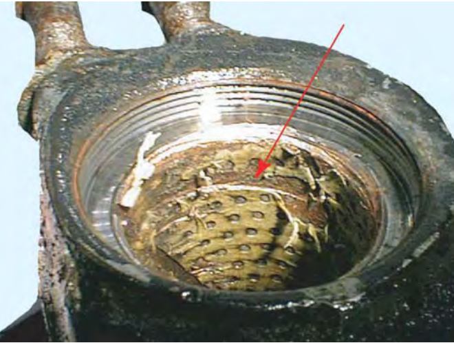
Improper Kingpin Installation
