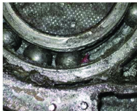
Release Bearing Failure
